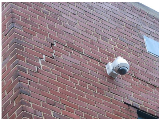
Cracked brick veneer at rear entrance
