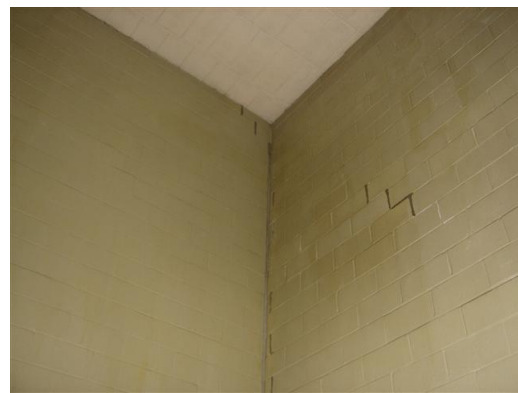
interior wall cracking
