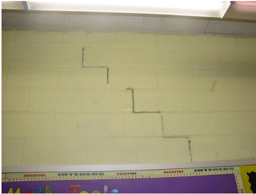
Interior Wall cracks
