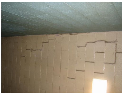
Interior wall cracking
