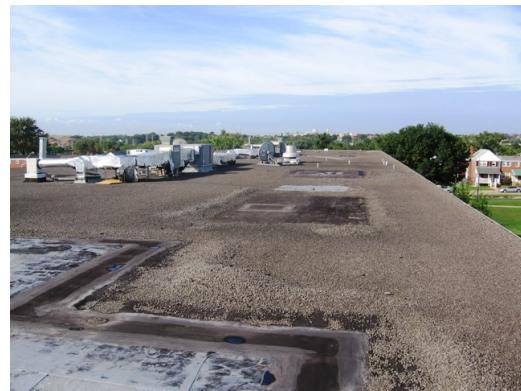
Roof with patches
