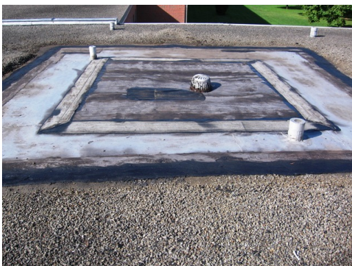
Patch at roof drain on main roof
