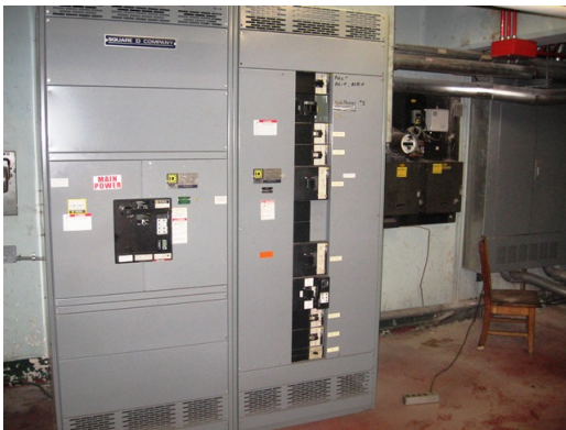
Main elec switchgear
