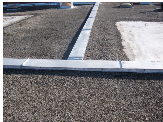
Metal expansion joint /coping cap
