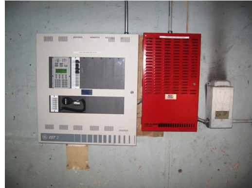
Fire alarm control panel
